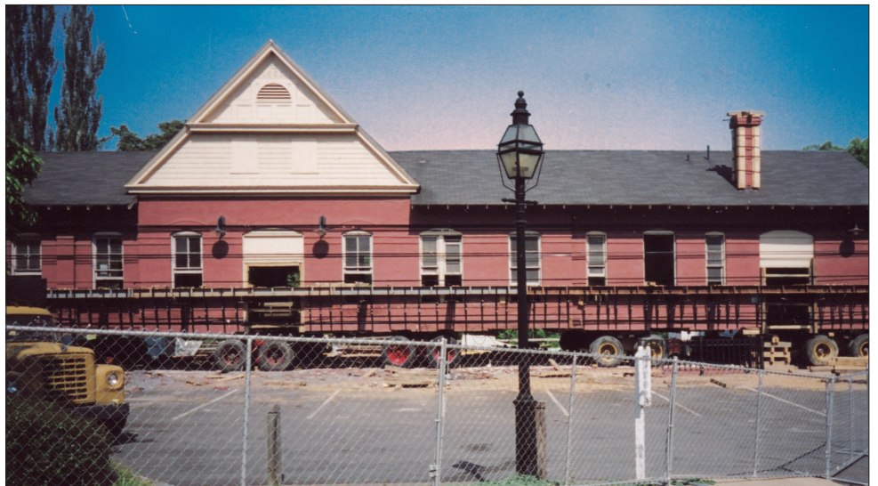
The simplest technology — wheel and board — moved the old train station to a new site.
